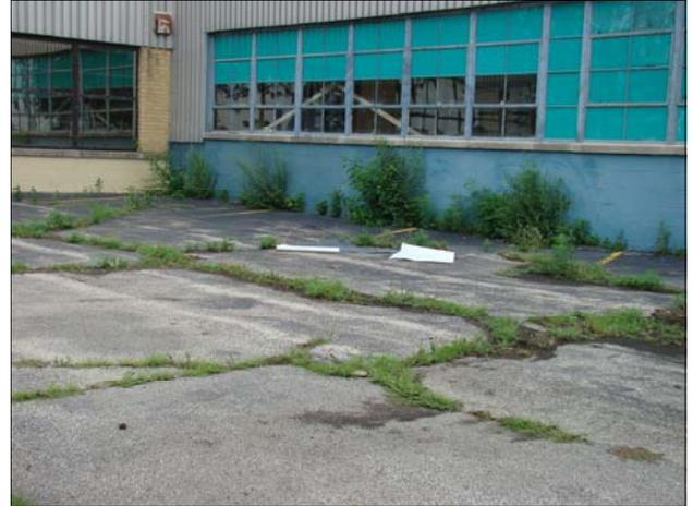
The front parking lot at Blaw-Knox Ingersoll Rand is dilapidated. Note weed growth through cracks in the parking lot and along the foundation.
