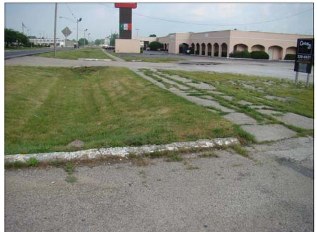
Portions of the sidewalk along Broadway East, such as the section shown above, are in need of repair or replacement due to severe cracking, settling and spalling concrete.
