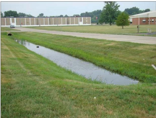
Storm water fills the open drainage ditch along the Armory Road right-of-way, evidence of inadequate drainage facilities.
