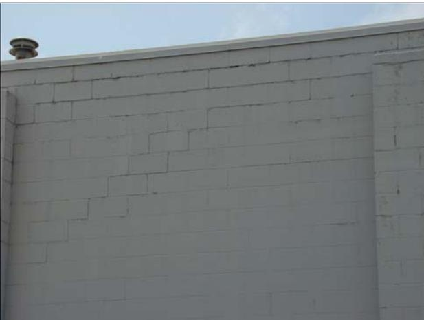
Step cracking on rear wall of Cross County Mall.
