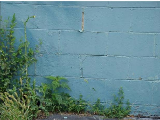
Deteriorated masonry wall of main Blaw-Knox Ingersoll Rand structure.
