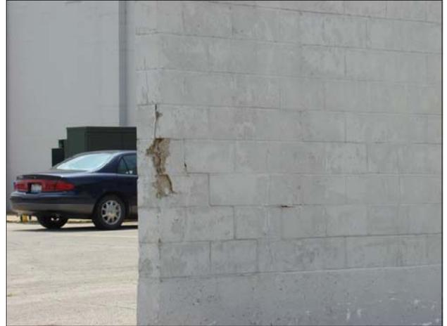
Deteriorated block wall adjacent to loading dock behind Cross County Mall.
