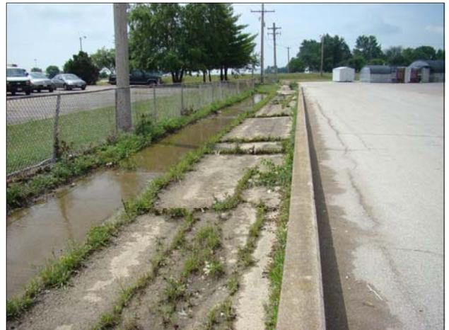
The drainage ditch running along the east side of the Cross County Mall property is deteriorated and inadequate.
