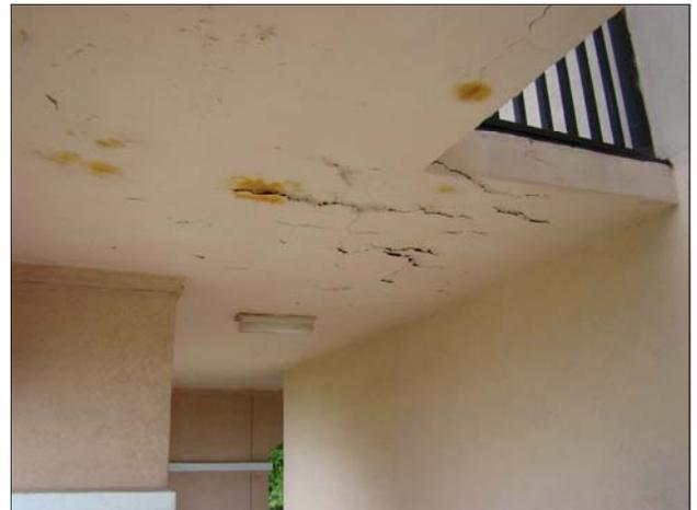
The ceiling at the Ramada Inn is cracking and peeling as a result of water damage.
