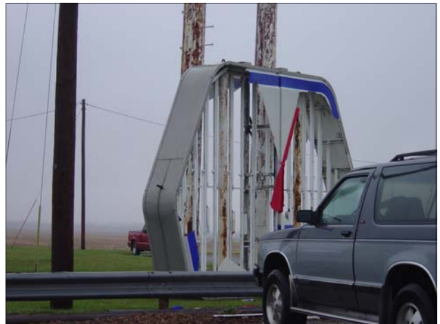
Broken Marathon Service Station sign. Note the rusted sign poles in the back.
